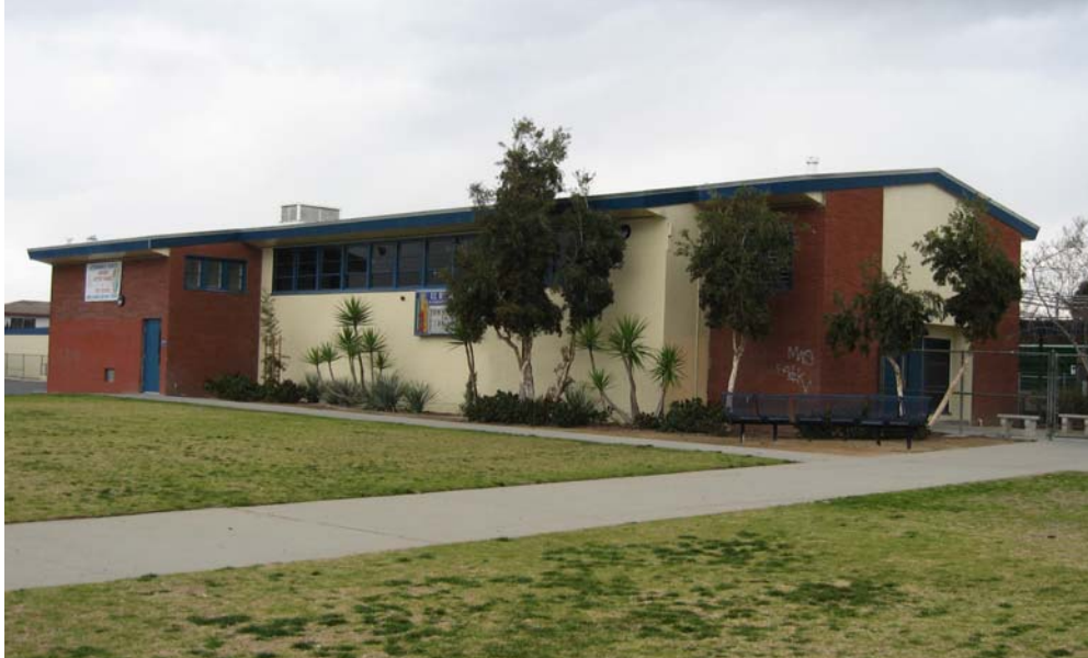
El Rancho Elementary School Multi-purpose Room as it looks today
